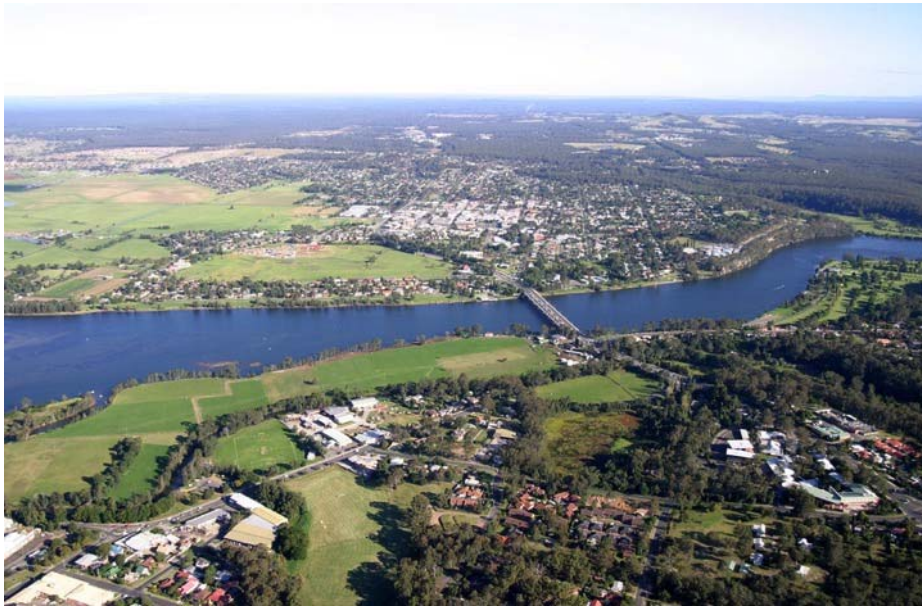
Source 3: Nowra Bridge, 2004, photographed by Daryl Jones
